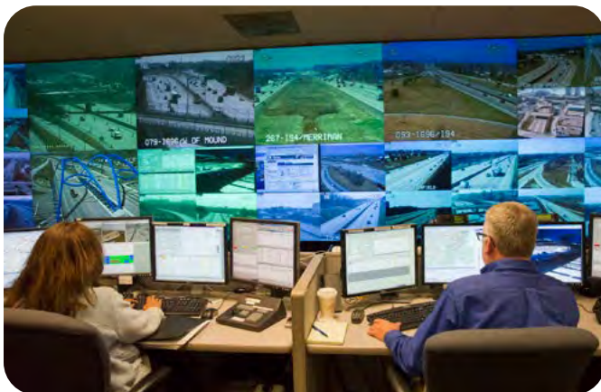
MDOT traffic operations center, Detroit
